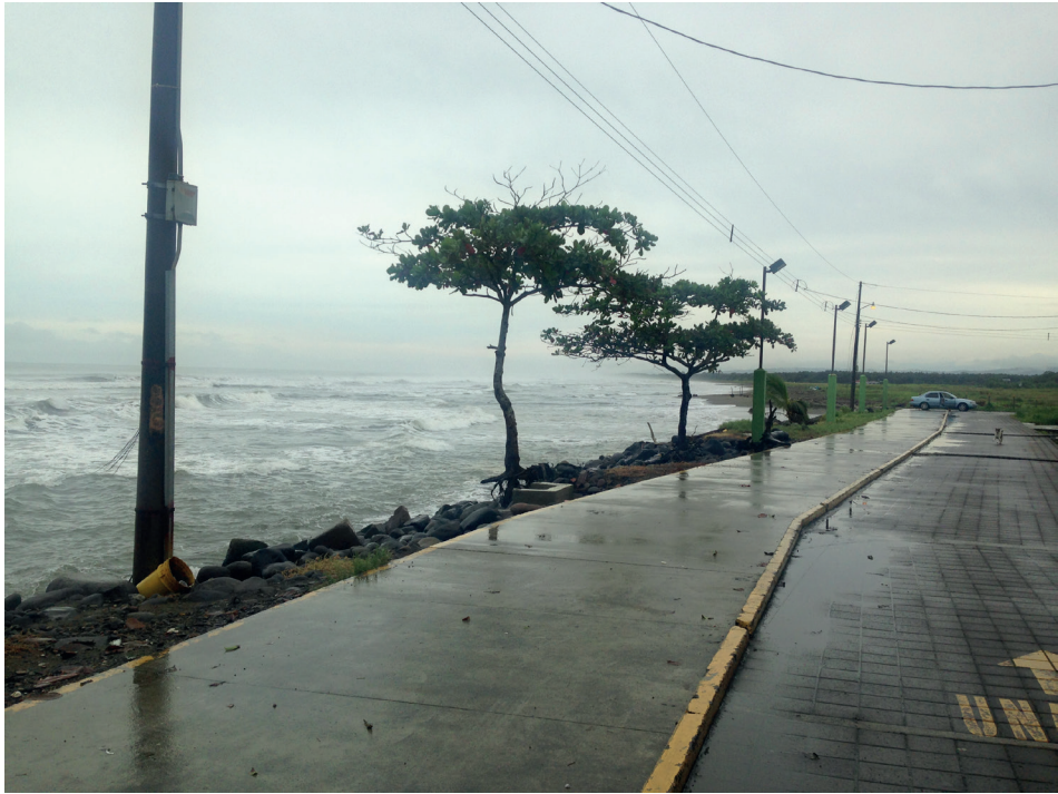
Figure 4. Placement of rocks for public infrastructure protection in Cieneguita Beach.
