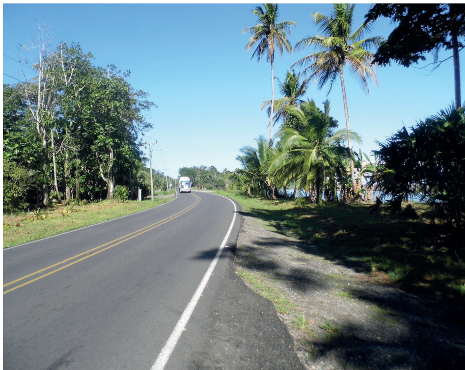
Figura 9. Proximity of the road with the beach erosion zone.
