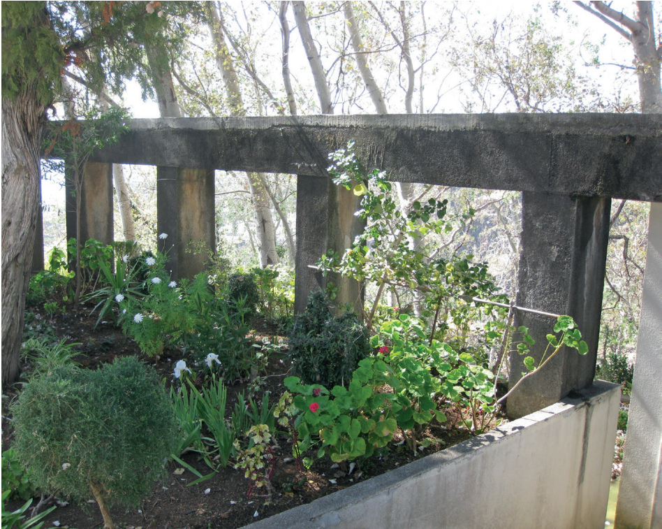
Figure 19. The bridge aqueduct along the west side of the praça at Lombada, with its concrete channel and piers.
