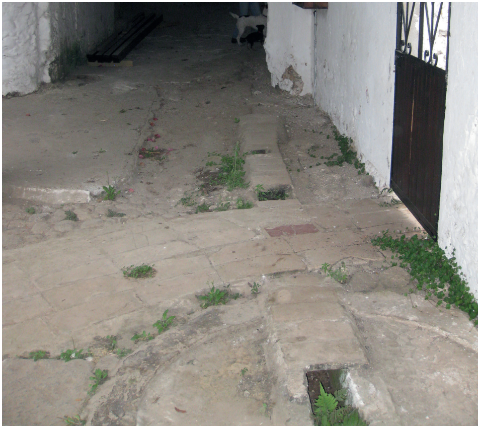
Figure 8. The mill chase at Hacienda de Pacho through which the turbines could be accessed. Water flowed out of the mill through the covered canal in the lower right.
