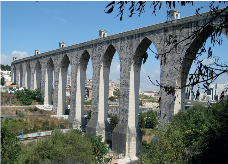
Figure 9. The Águas Livres aqueduct bridge in Lisbon with its unusual Gothic arches.
