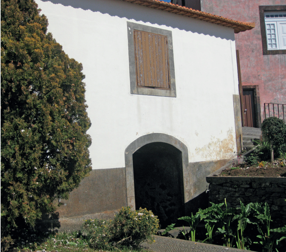
Figure 17. The downslope side of the mill structure at Lombada, Madeira. Evident are the chase below (compare with Figure 8) and the shuttered window on the second level where the millstones are located.
