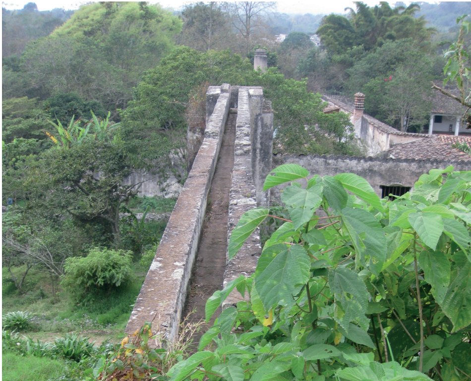
Figure 4. View along the top of the aqueduct that carried water from the spring to the mill
