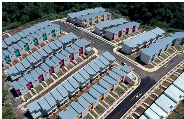
Figure 2. Aerial view of the Shikaba Residential Residential Project
