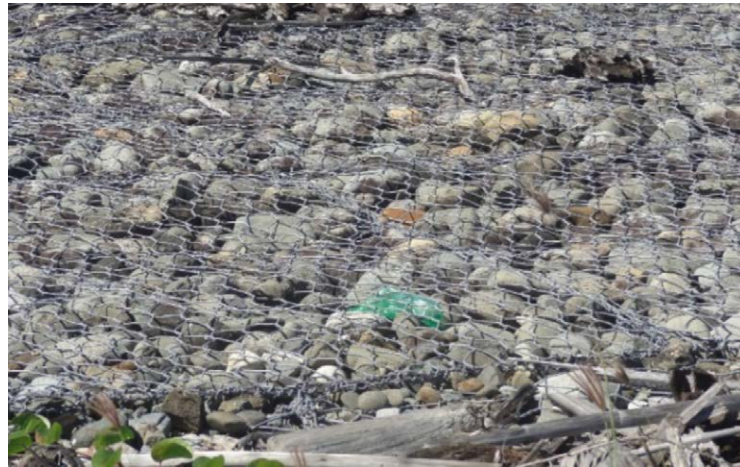
Figure 2. Airport Sector: Installation of gabions. Taken in the field on December 6, 2017.
